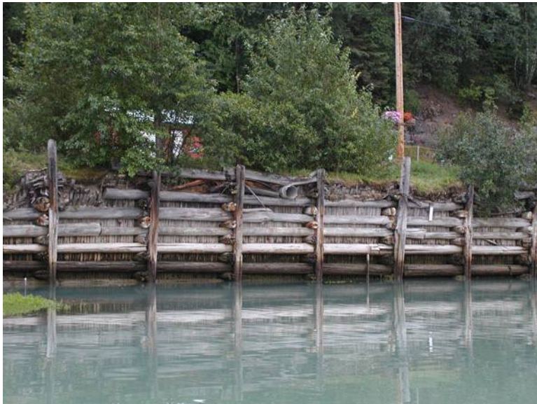
Figure 2-4. Crib wall at Railroad Dock. This crib wall, although it is not itself historic, shows the historical method that was used to construct this wharf out into the harbor, and is an example of a construction method that is similar to the method used to build the original Moore's Wharf before and during the Gold Rush era, as described by Captain Moore. Seen from Small Boat Harbor (July 2004).
