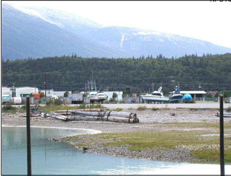
Figure 2-6. Old pilings discarded on the beach. West side of the Small Boat Harbor. It is not clear in which era these pilings were built, but they represent, in general, the methods of wharf construction that date back to Skagway's early years (July 2004).
