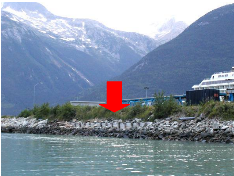
Figure 2-5. Crib wall remnant visible on west side of Small Boat Harbor, partially obscured by rip rap (loose rock fill) (July 2004).
