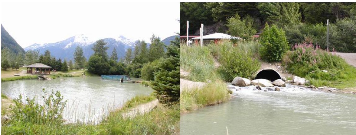
Figure 2-12. (Left) Fish pond along Pullen Creek, and (right) Creek emerging from culvert under road to Railroad Dock into pond.
