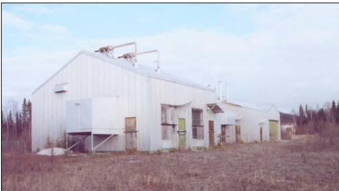
Figure 41. Timber Pump Station, May 2002. From collection of USARAK.
