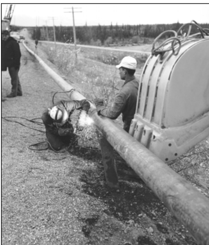
Figure 7. Pipe welding. NARA, DA 573 #373.
