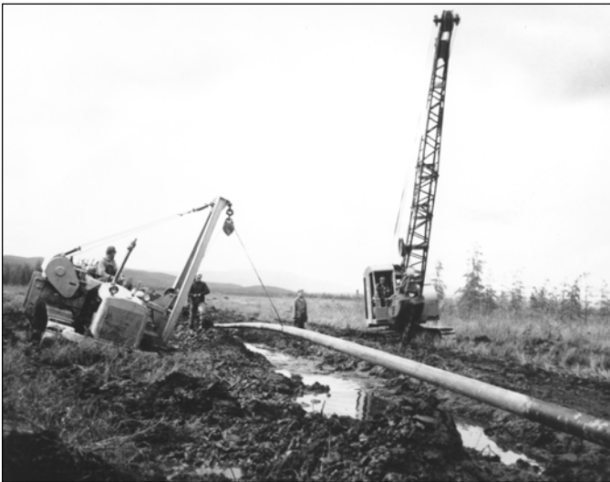
Figure 6. Pipeline construction. NARA.
