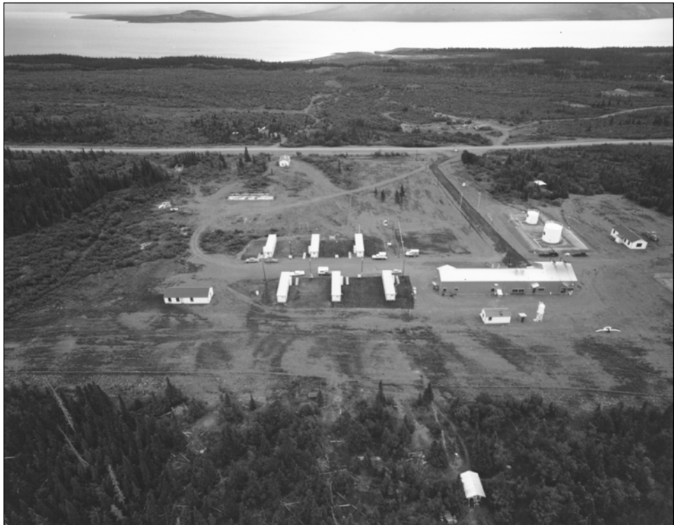
Figure 34. Destruction Bay Pump Station. NARA.
