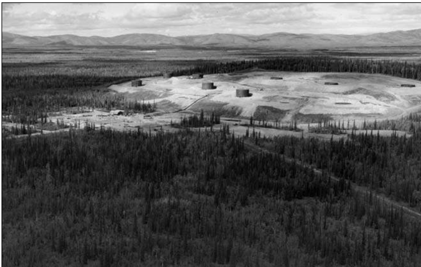
Figure 9. Tok terminal under construction, 1954. NARA.
