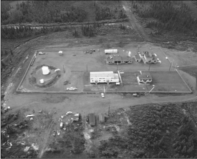
Figure 18. Donjek Pump Station. NARA.
