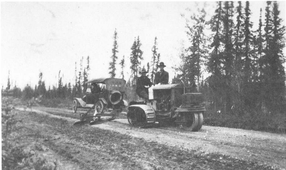
Tractor pulling grader on newly graded road, 1930s. Alaska Road Commission Collection, AHL.
