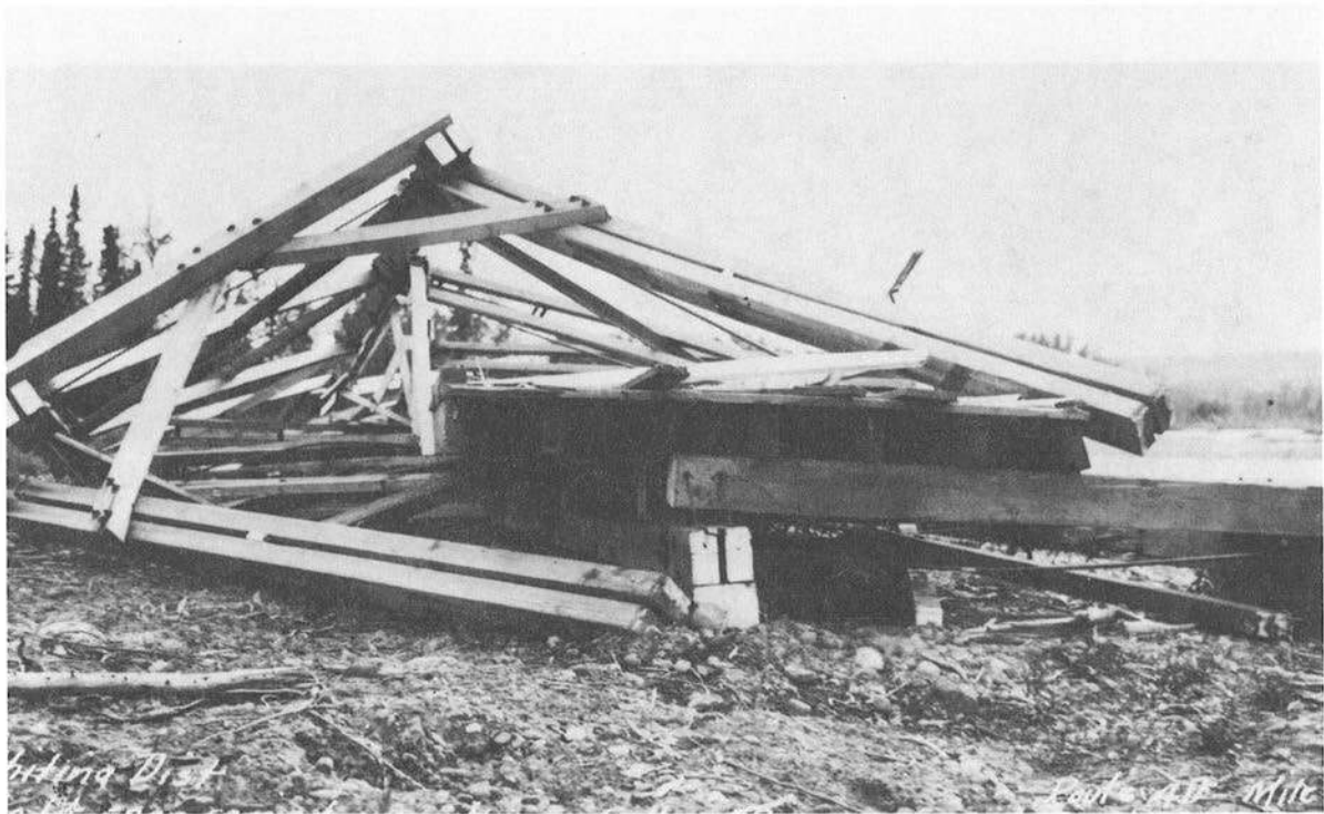
Bridge, with 100-foot span over the Gulkana River, at mile 128, Richardson Highway, was carried away by ice, May 9, 1933. Ray Huddleston Collection, UAF.
