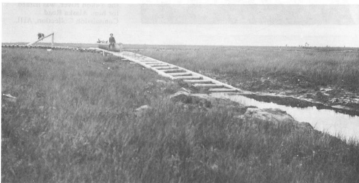
Dam, rollers, cavel and winch between two lakes on the Yukon-Kuskokwim Portage. Alaska Road Commission Collection, AHL.
