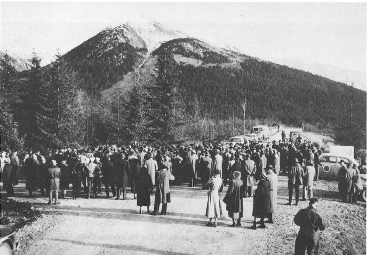
Seward Highway completed at Girdwood, 1951. Alaska Railroad Collection, AMHA.
