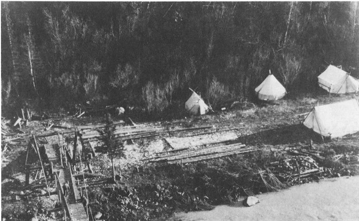
Aerial view of Alaska Road Commission camp and bridge construction on the Richardson Highway, 1930s. Ray Huddleston Collection, UAF.
