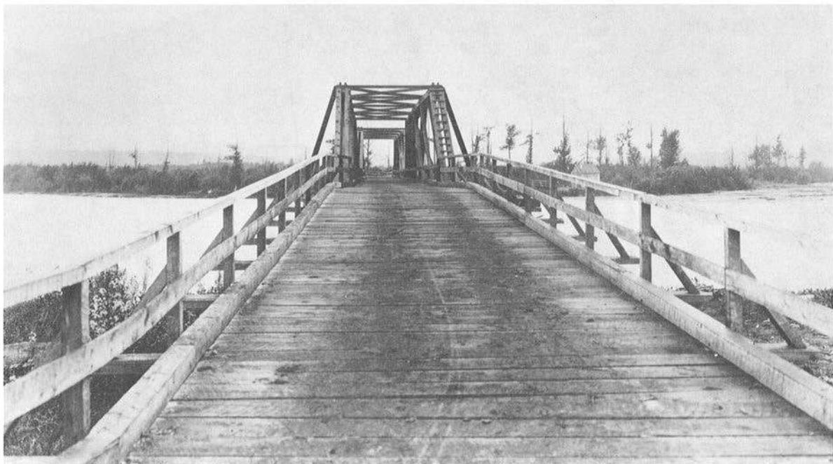
Tazlina River bridge, about 1909-1919. Francis E. Pope Collection, UAF.
