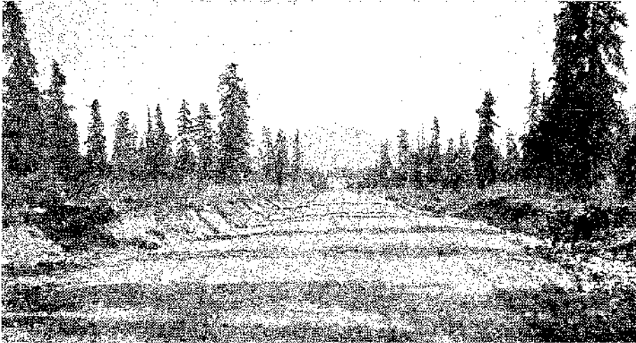
COMPLETED GRAVEL ROAD---SOUTHWESTERN DISTRICT
