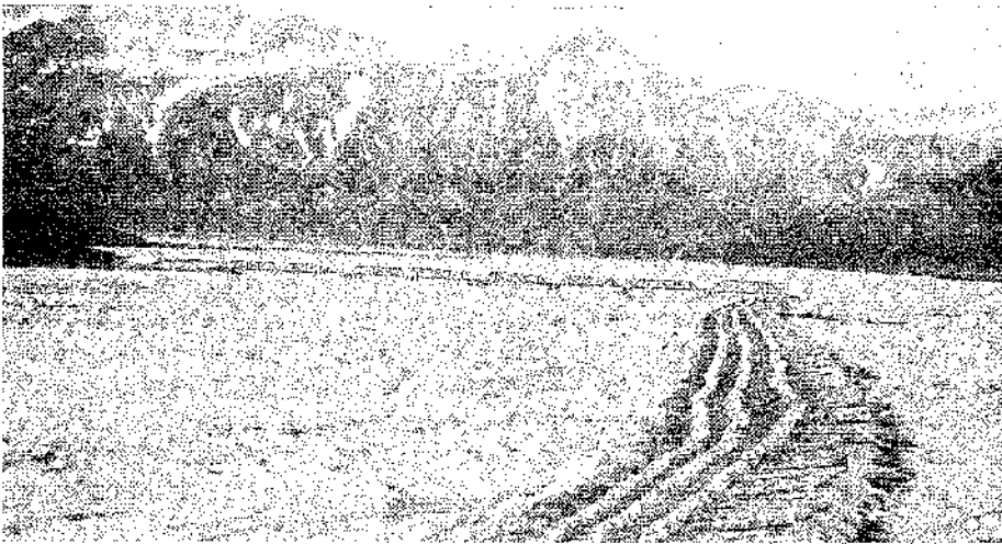
A WANDERING GLACIAL STREAM CONFINED TO HALF ITS NATURAL BED IN ORDER TO REDUCE BRIDGE REQUIREMENTS
