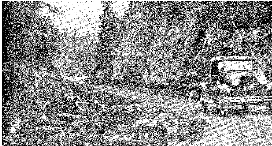
RICHARDSON HIGHWAY NEAR TIEKHELL
