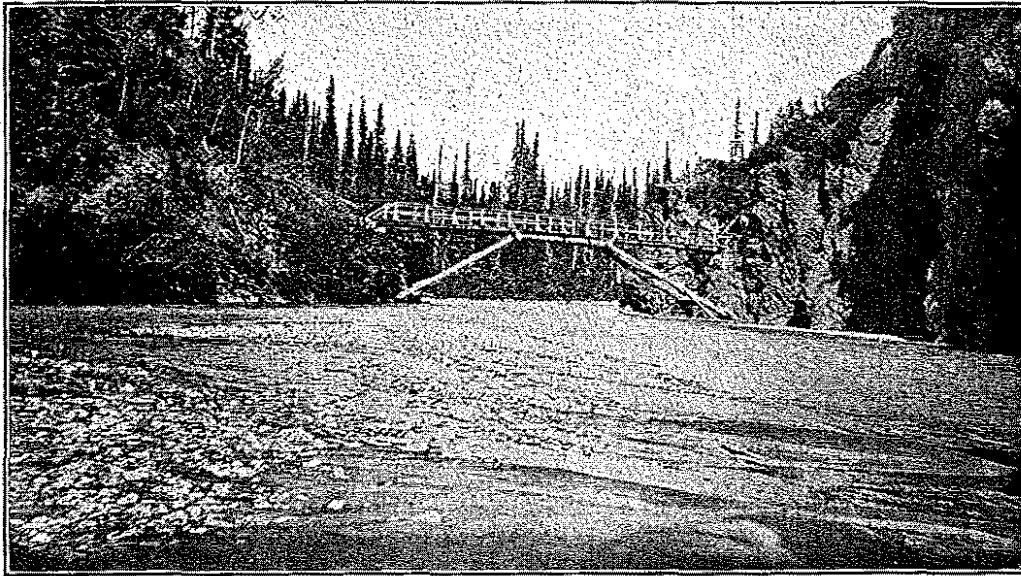
BULL RIVER BRIDGE, PACK TRAIL
