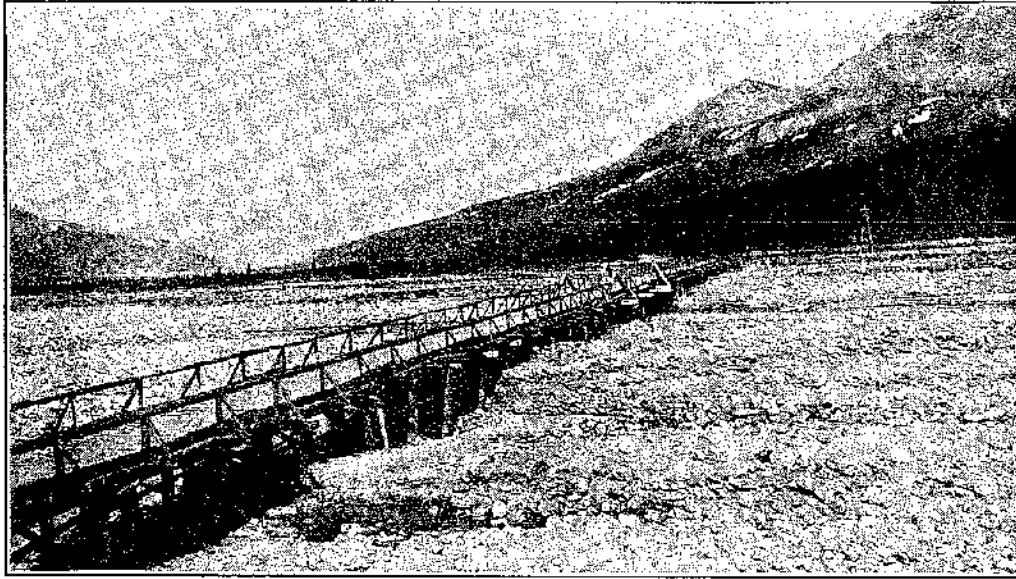
TRESTLE ACROSS GLACIER STREAM NEAR MILLERS, MILE 230, RICHARDSON HIGHWAY.
