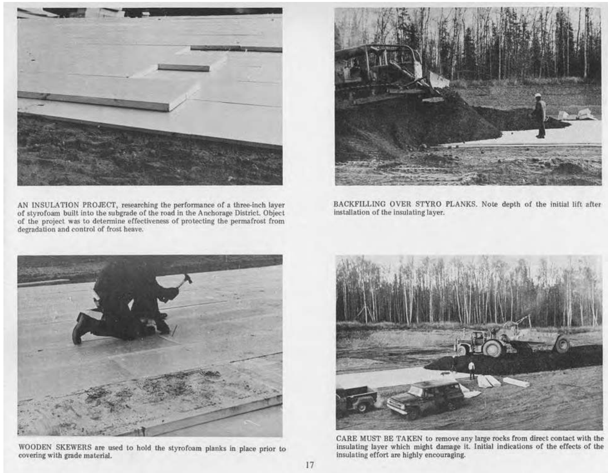
Figure 26. Styrofoam subgrade insulation installation. Source: ADH Annual Report, 1969.
