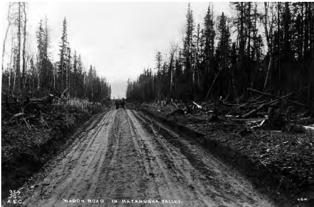
Figure 20. Wagon Road in the Matanuska Valley. Example of a wagon road with an earth surface, 1918. Source: H.G. Kaiser, Alaska Railroad Collection; Anchorage Museum, B1979.002.G959.
