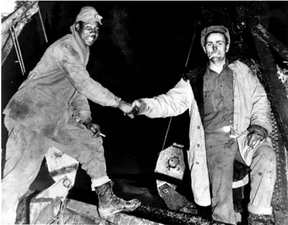
Figure 13. Photograph of Corporal Refines Sims, Jr. (left) and Private Alfred Jalufka (right) shaking hands upon meeting to close the final gap of the Alaska Highway in 1942. Photograph from U.S. Army Corps of Engineers.
