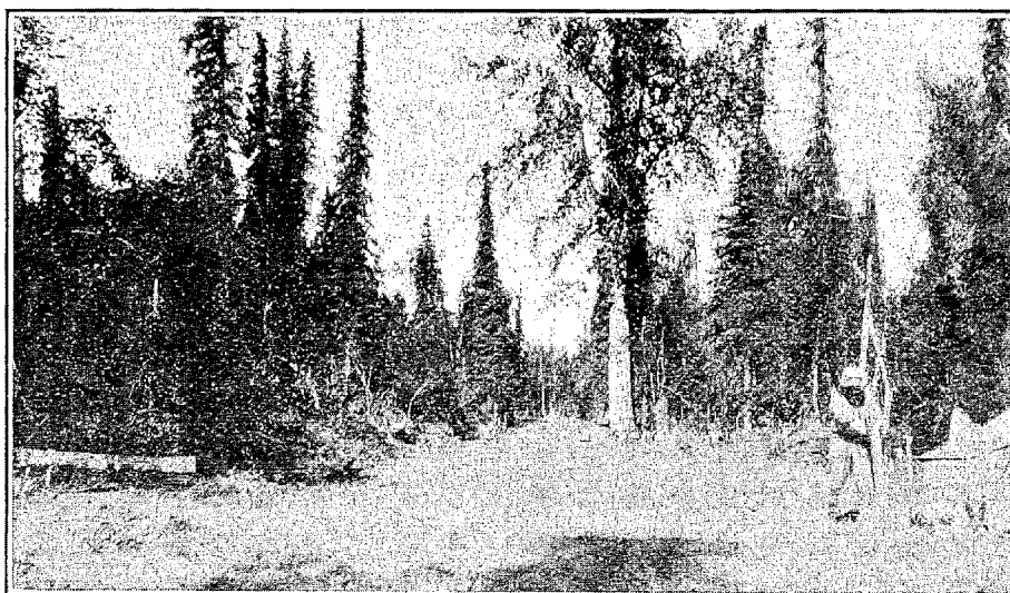
CLEARING TALKEETNA-CACHE CREEK ROAD.
