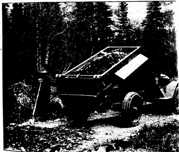
PLACING SURFACING NEAR CHITINA, RICHARDSON ROAD.
