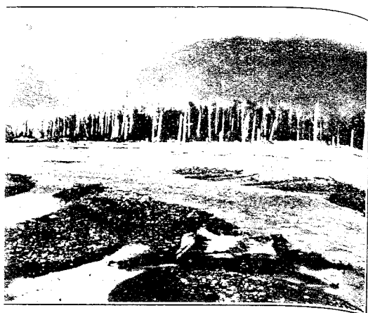
ONE MILE 1 ON VALDEZ-FAIRBANKS ROAD.
