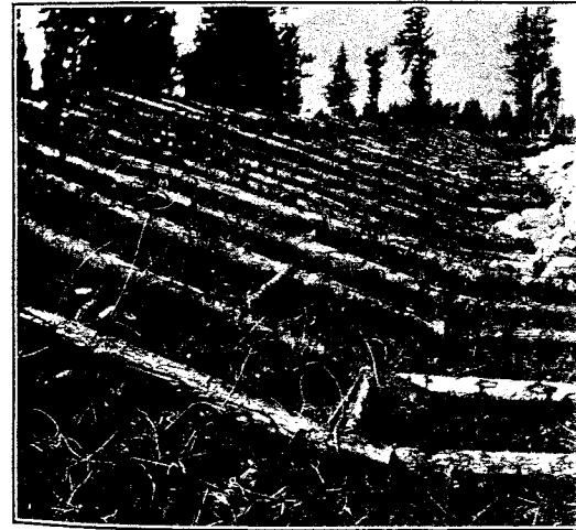
VALDEZ DIKE EMBANKMENT SHOWING F
