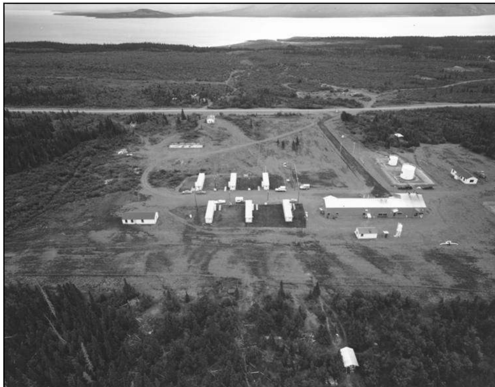
Figure 34. Destruction Bay Pump Station. NARA.
