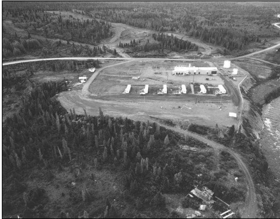
Figure 33. Blanchard River Pump Station. NARA.
