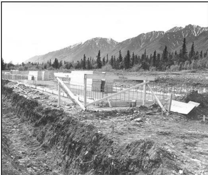
Figure 32. Destruction Bay under construction. NARA.
