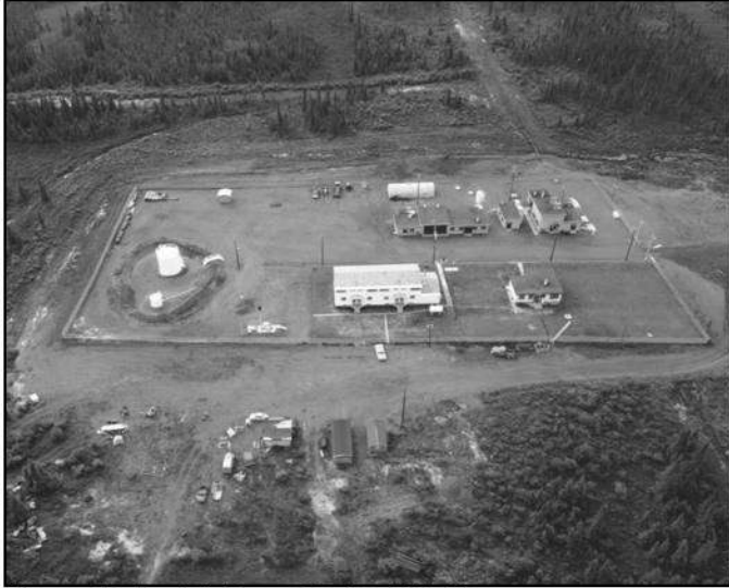
Figure 18. Donjek Pump Station. NARA.
