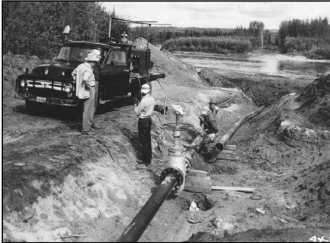
Figure 5. Laying pipe for underwater crossing. NARA, A4-3826.
