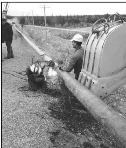
Figure 7. Pipe welding. NARA, DA 573 #373.
