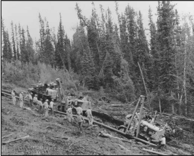
Figure 11. Haines-Fairbanks Pipeline construction. NARA.
