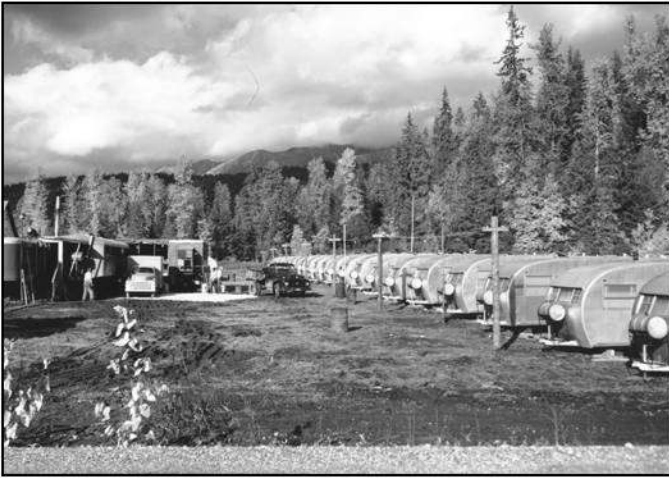
Figure 10. 24 Sept 1954. Contractor's Camp at Mosquito Lake 25 miles from Haines. NARA.
