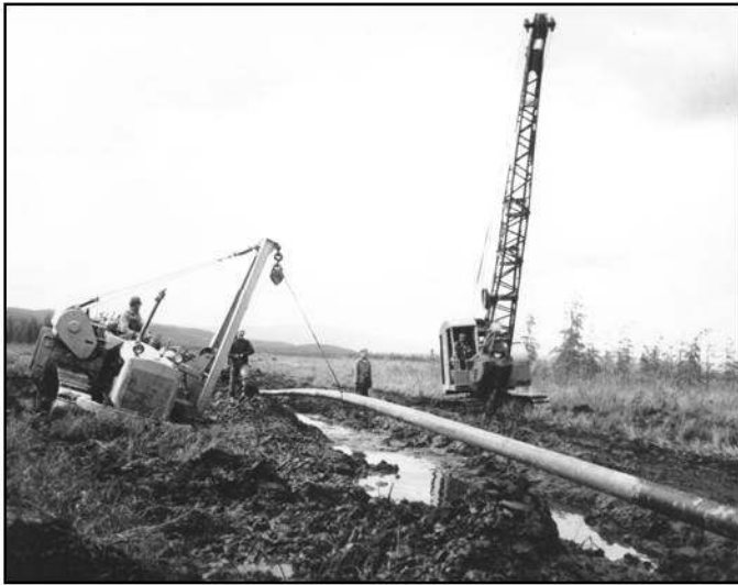
Figure 6. Pipeline construction. NARA.
