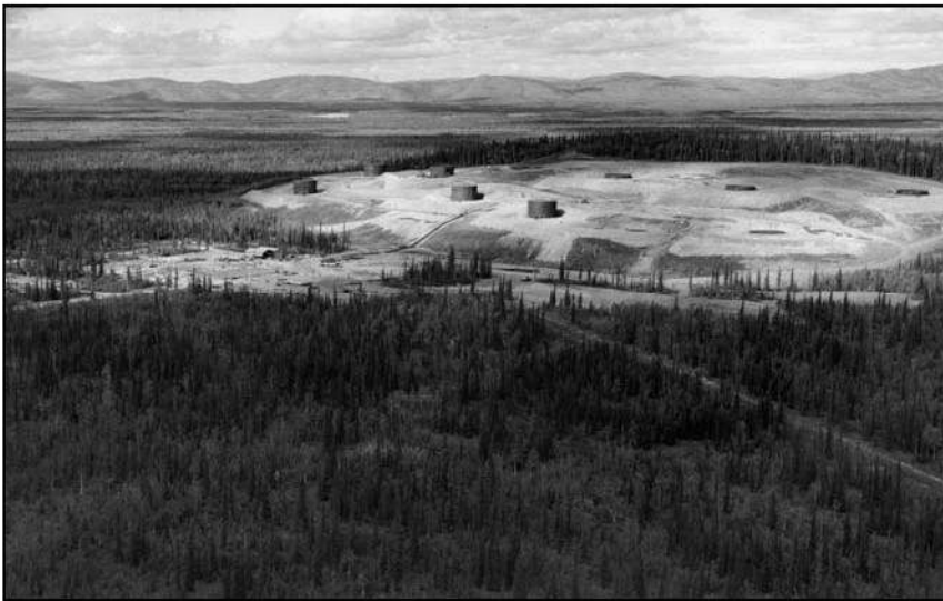
Figure 9. Tok terminal under construction, 1954. NARA.
