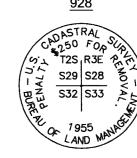
T2S R3F FM CORNER OF SECS 29, 28, 32, & 33 FOUND 3 1/4" BRASS CAP ON 2 1/2" IRON POST, 0.5' ABOVE GRADE GOOD CONDITION
