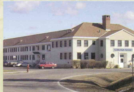
Murphy Hall, originally BOQ, bachelor officers' quarters. USAG-AK cultural resources program.
