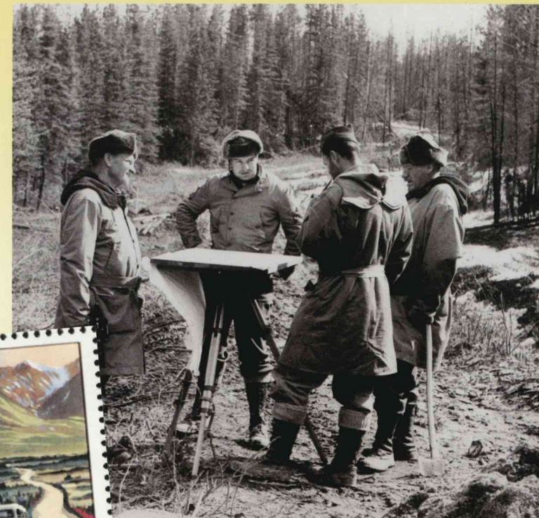
Above: A team of U.S. Army Engineers lay out the pioneer road – the road that became the Alaska Highway in 1942. UAFairbanks Archives, 1992-0077-00203.
