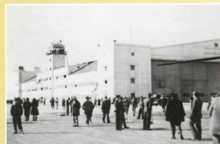
Hangar One at Ladd Field. UAF Archives, Cecil H. Kornegay Collection, 1999-0204-00045.
