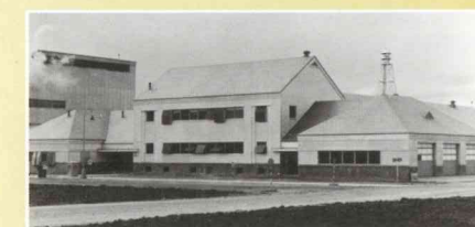
Quartermaster building and the adjacent power plant. AAF photo.
