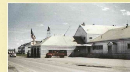
Ladd Field Fire House (and Rescue Unit), north side of Quartermaster building. UAF Archives, Cecil H. Kornegay Collection, 1999-204-112
